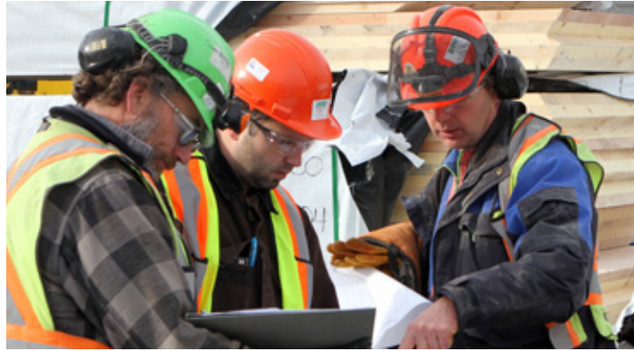
Design-Build team collaborating during construction.
