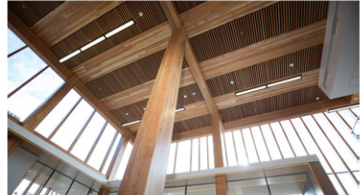
Glulam columns and beams in the main foyer.
