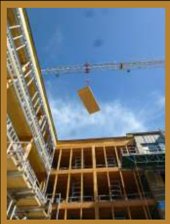
UBC ESSB Stair install
